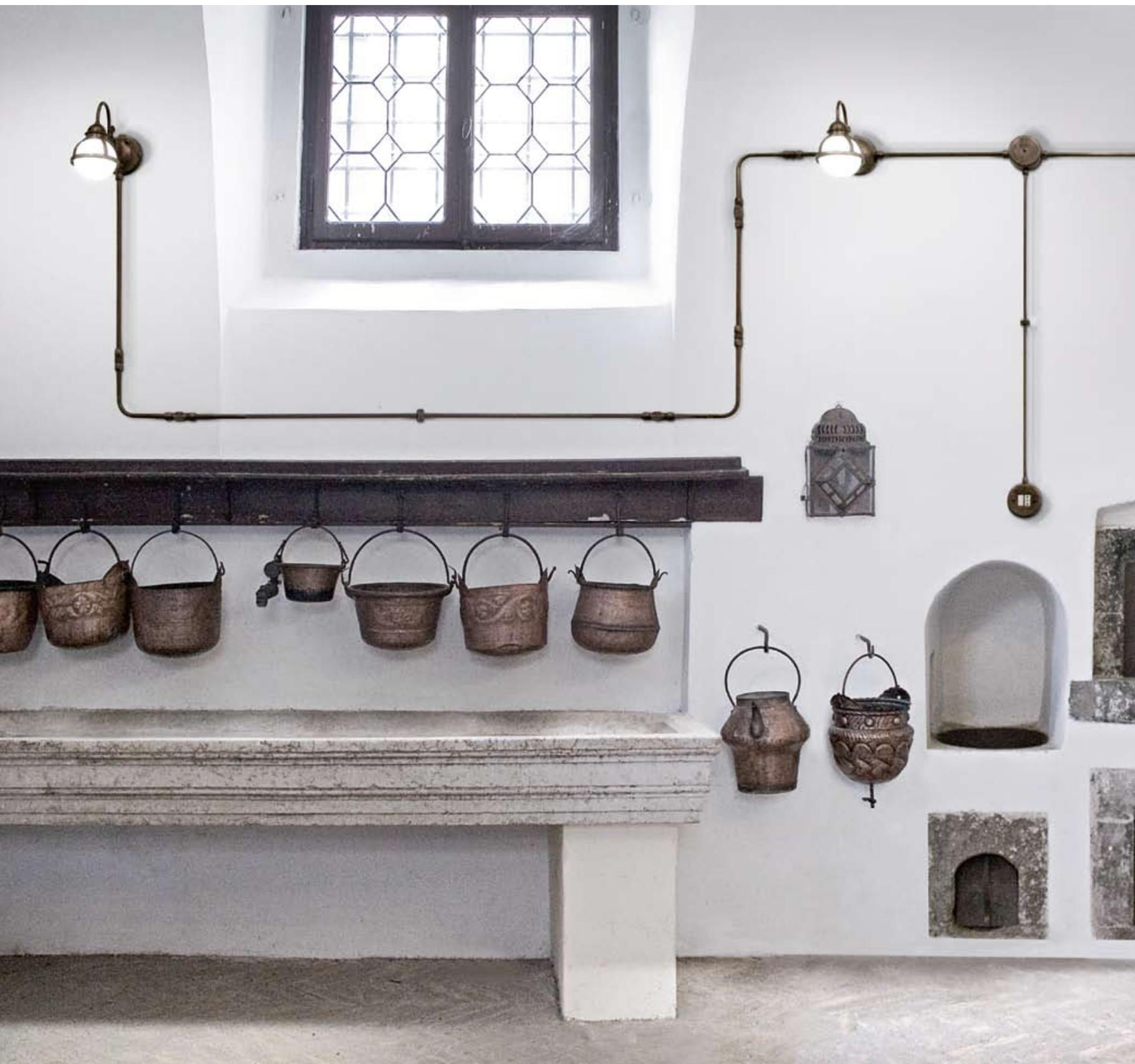
This solution develops the previously proposal for the outdoor electric installation with cable and ceramic components as switches, insulators and plugs.
